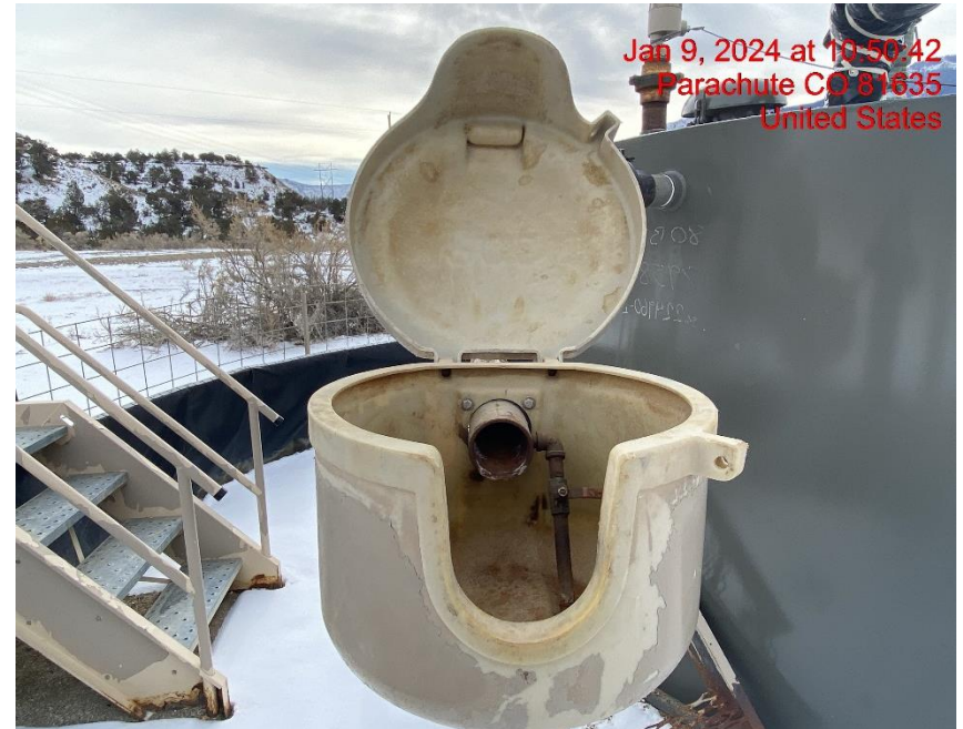
Open-Ended Load Line – Photo #08641
