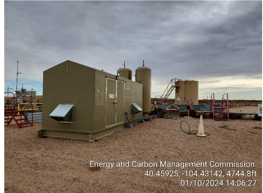
Photo 2 – Instrumental Air Compressor Unit
