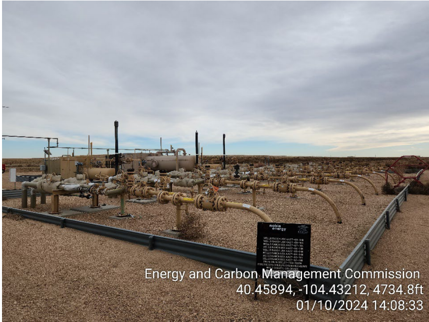
Photo 7 – Separators and Headers
