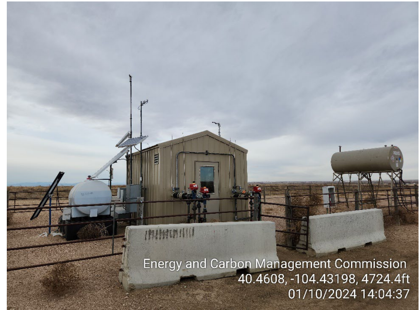
Photo 4 – Gas Lift Injection Meter House and Methanol Day Tank
