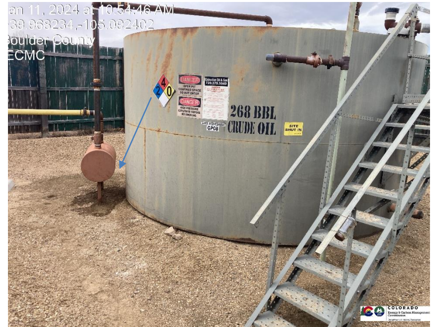
Pic 2 stained soil / leak near tank
