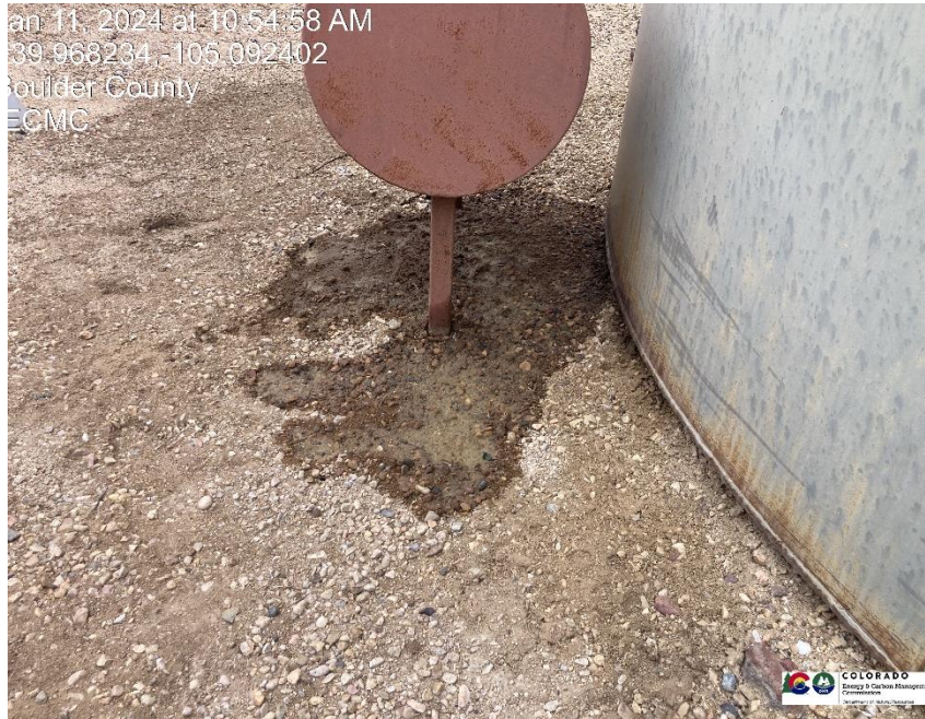
Pic 3 Stained soil / leak
