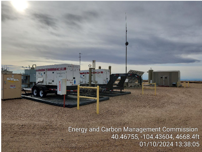
Photo 9 – Generators and Instrumental Air Unit
