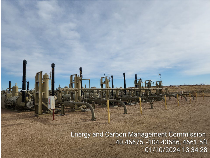
Photo 3 – West Separators and Sand Traps
