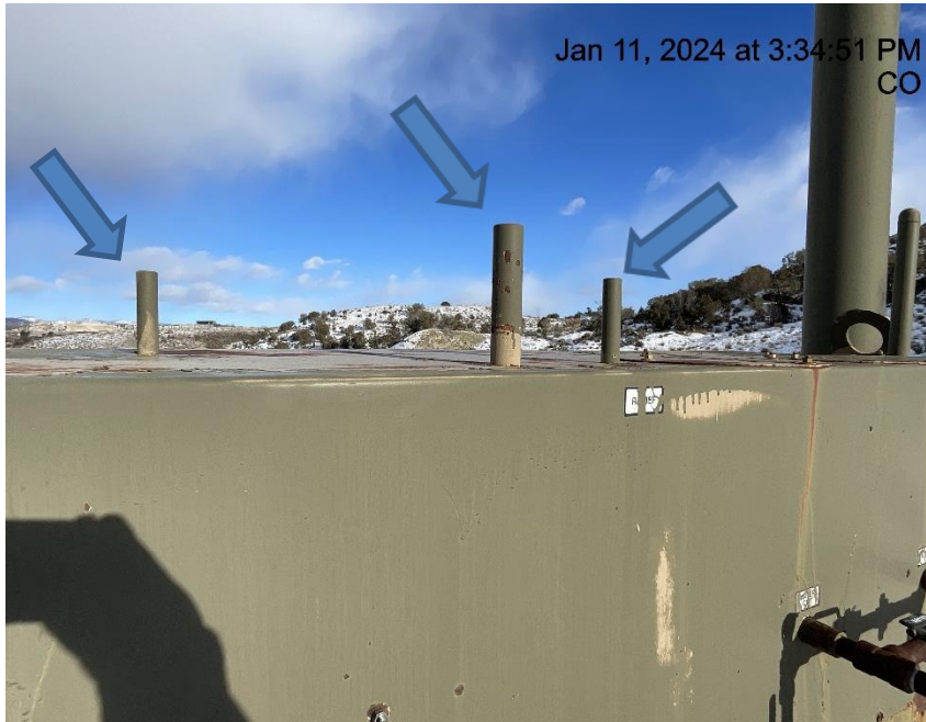
Photo # 2673 PRV & rupture disc vent lines lack caps
