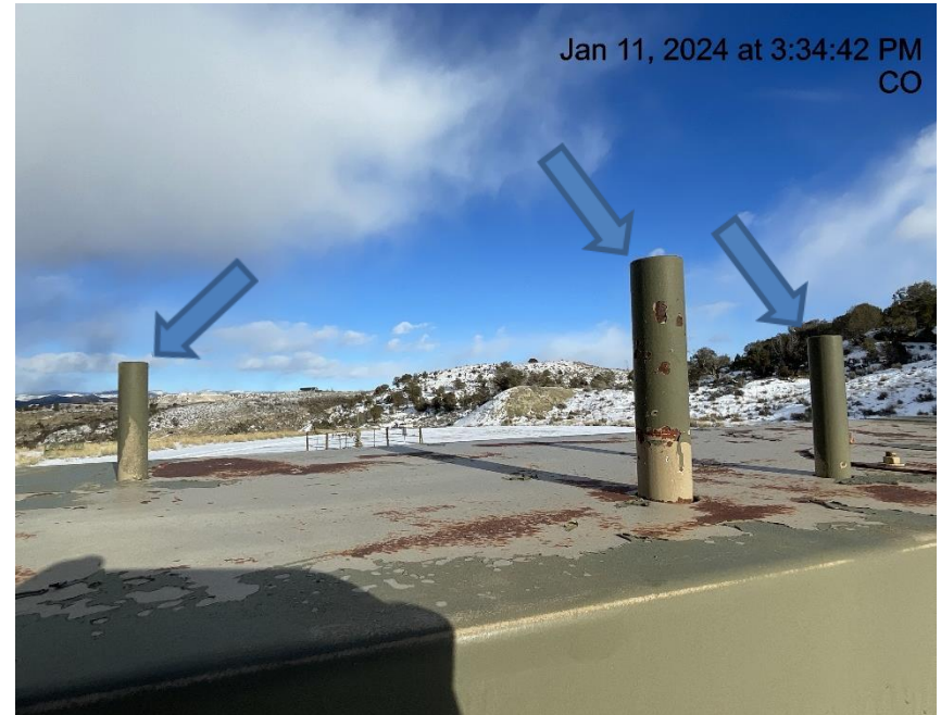
Photo # 2674 PRV & rupture disc vent lines lack caps
