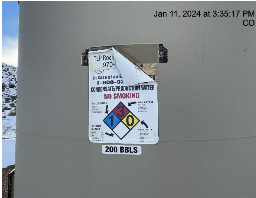
Photo # 2675 Tank label losing adhesion
