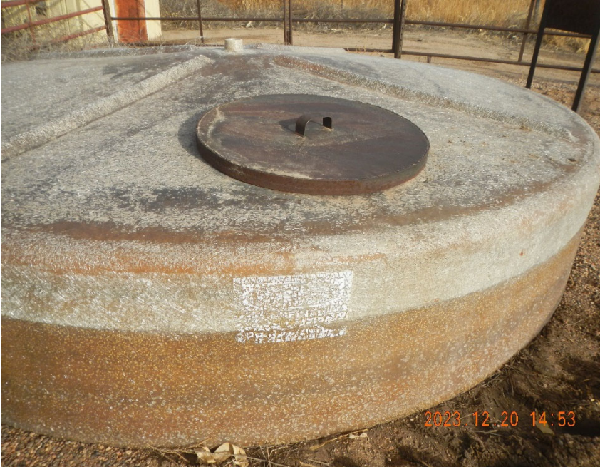
7. Unreadable Content/Quantity/Hazard label on tank.
