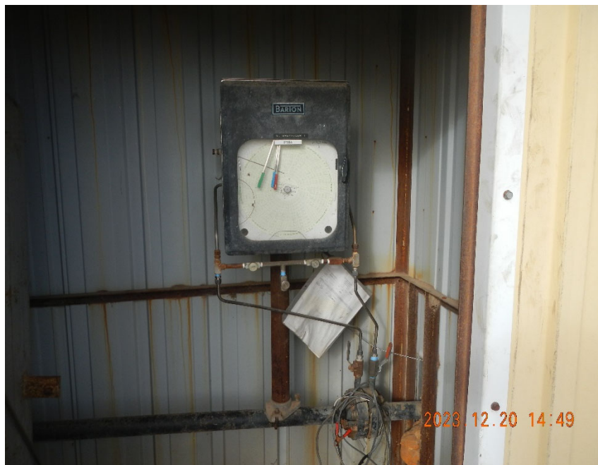
5. Gas meter inside meter shed.
