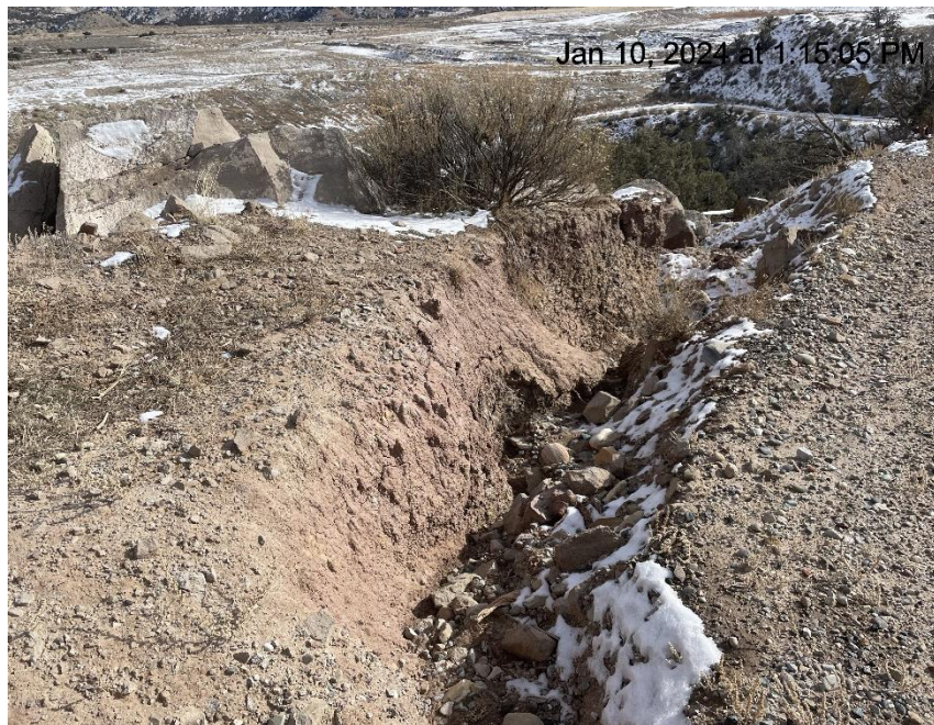
Photo # 2316 Erosion & transport of sediment/insufficient runoff controls/BMP's (lease road near entrance to location)
