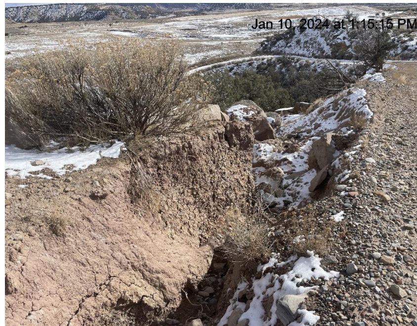
Photo # 2317 Erosion & transport of sediment/insufficient runoff controls/BMP's (lease road near entrance to location)
