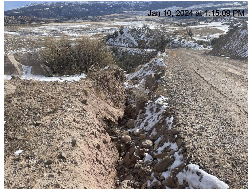
Photo # 2315 Erosion & transport of sediment/insufficient runoff controls/BMP's (lease road near entrance to location)
