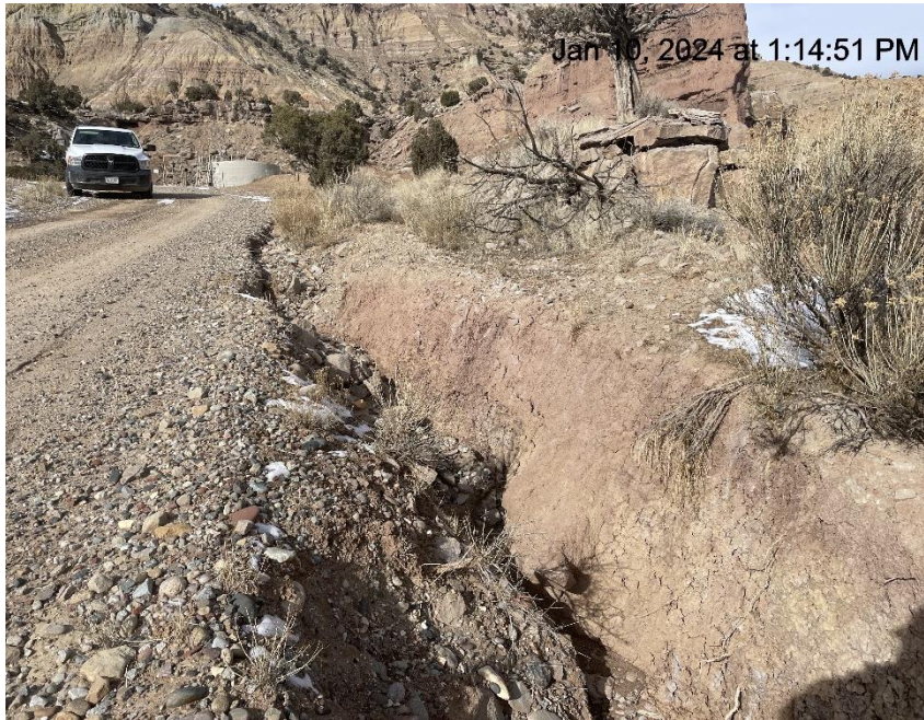
Photo # 2314 Erosion & transport of sediment/insufficient runoff controls/BMP's (lease road near entrance to location)
