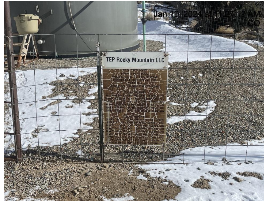
Photo # 2267 Battery sign weathered/cracking/damaged & illegible
