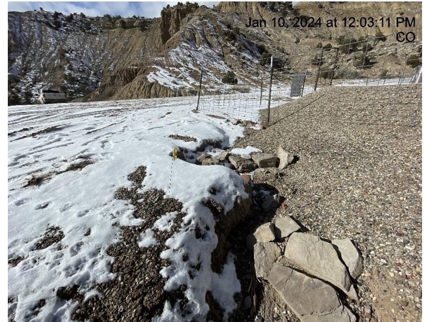
Photo # 2273 Check dam needs maintenance
