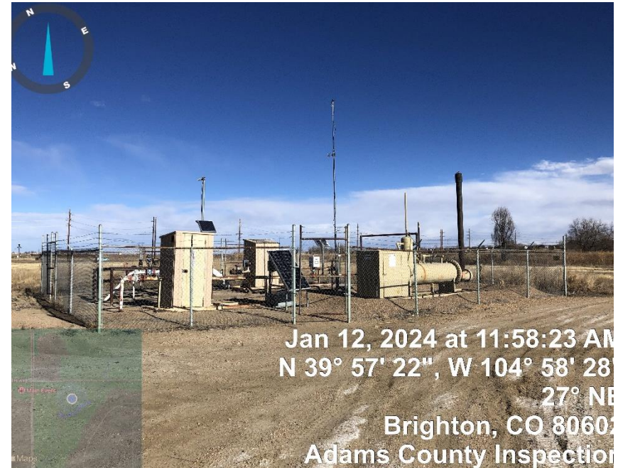
Photo#2 Separator/Automation RTU/(2) Gas Meters
