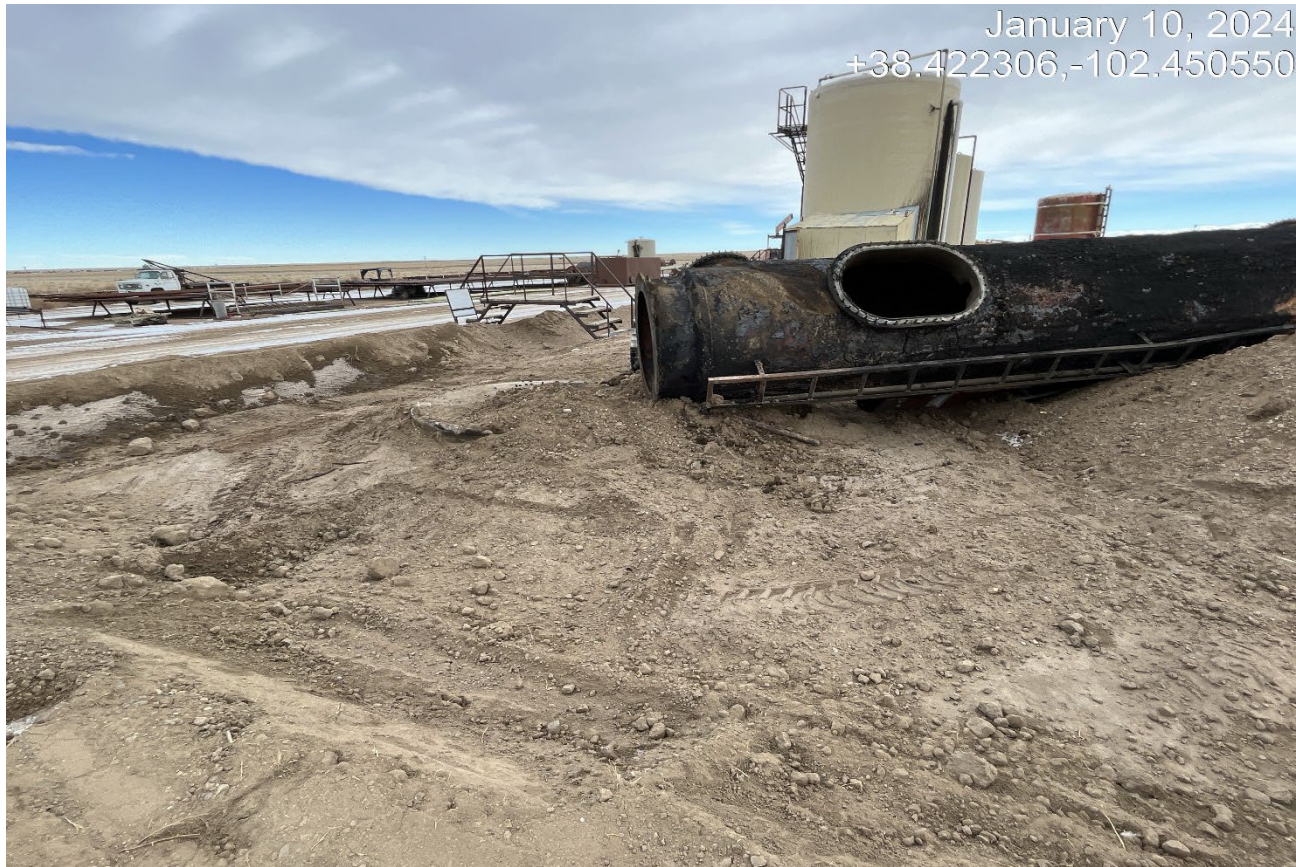
Photo 7. Facing northeast toward the heater treater which was burned during a recent fire. The treater has since fallen over and needs to be removed if it is no longer functional.
