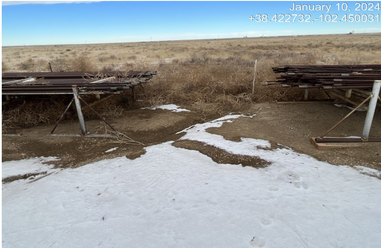
Photo 17. Facing toward the north central side of the location. There is an erosion channel beginning to develop in this area which is transporting sediment offsite.
