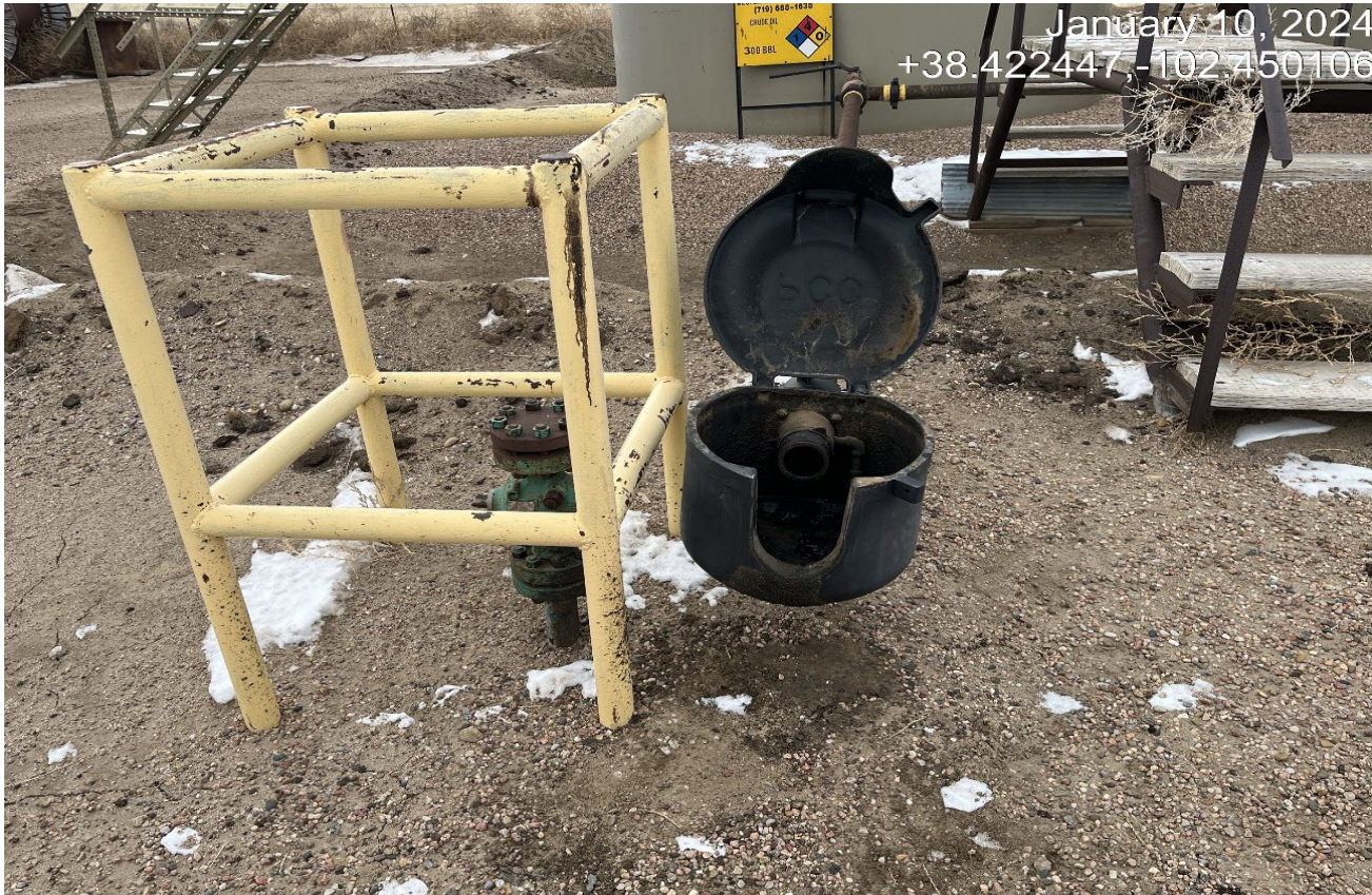
Photo 5. There is oil stained soils at the pipe outlet which is not in containment and the lid was left open.
