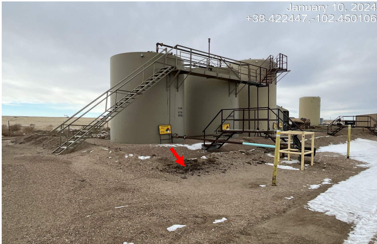
Photo 4. Facing toward the PYLES offsite tank battery at the location. Stained soil was removed from the outlet area. There is hardened hydrocarbon substances shown at red arrow.
