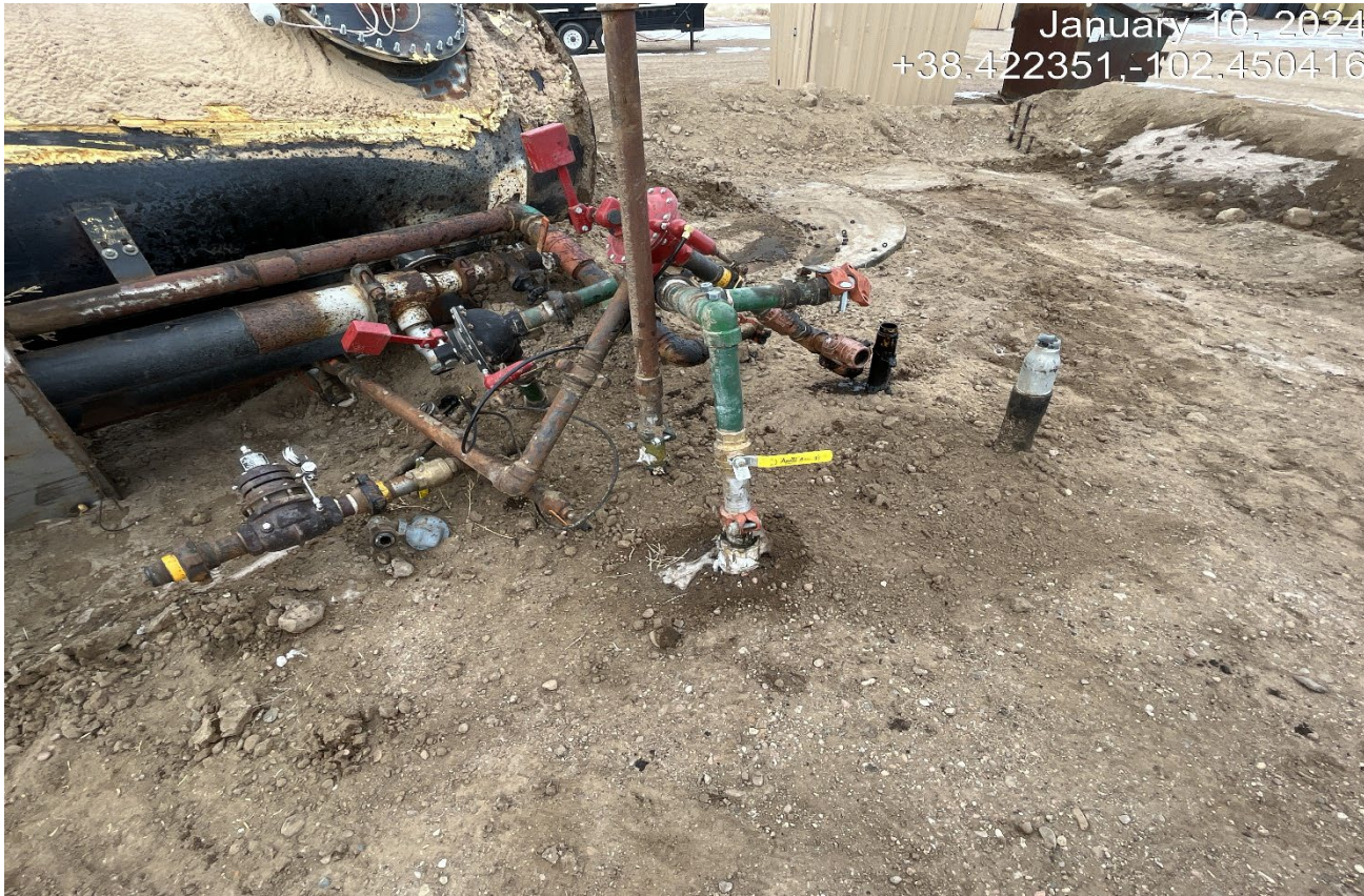
Photo 8. There is oil stained soils at the pipe connections where the treater fell over.
