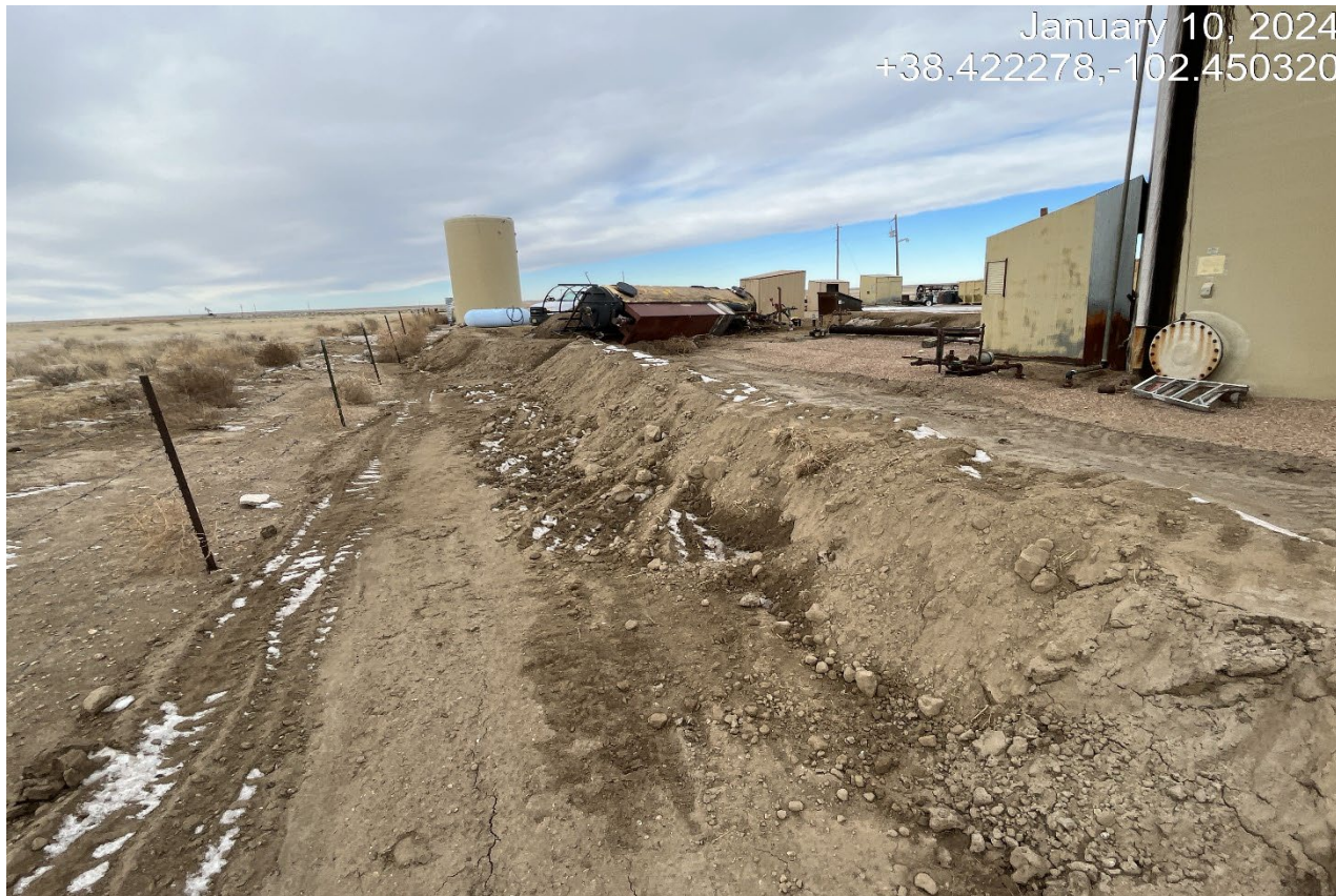
Photo 9. Facing west at the south side of the location and backside of the tank battery. The berms around the tank battery are not compacted for impermeability.
