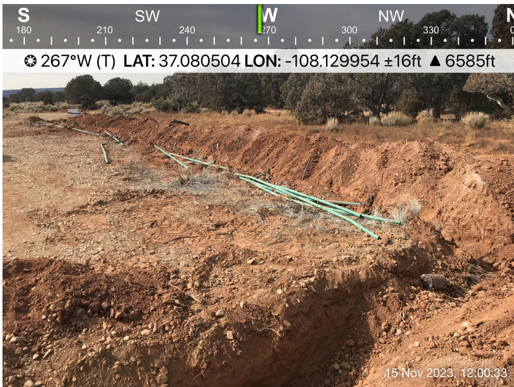
Photo 4: Overall flowline excavation, 11/15/2023.
