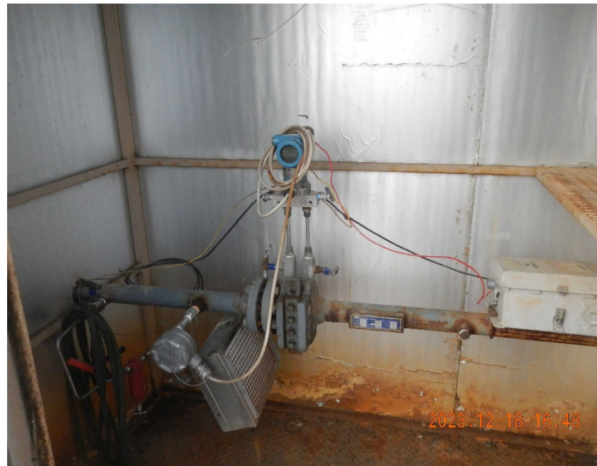
6. Digital gas meter inside meter shed.
