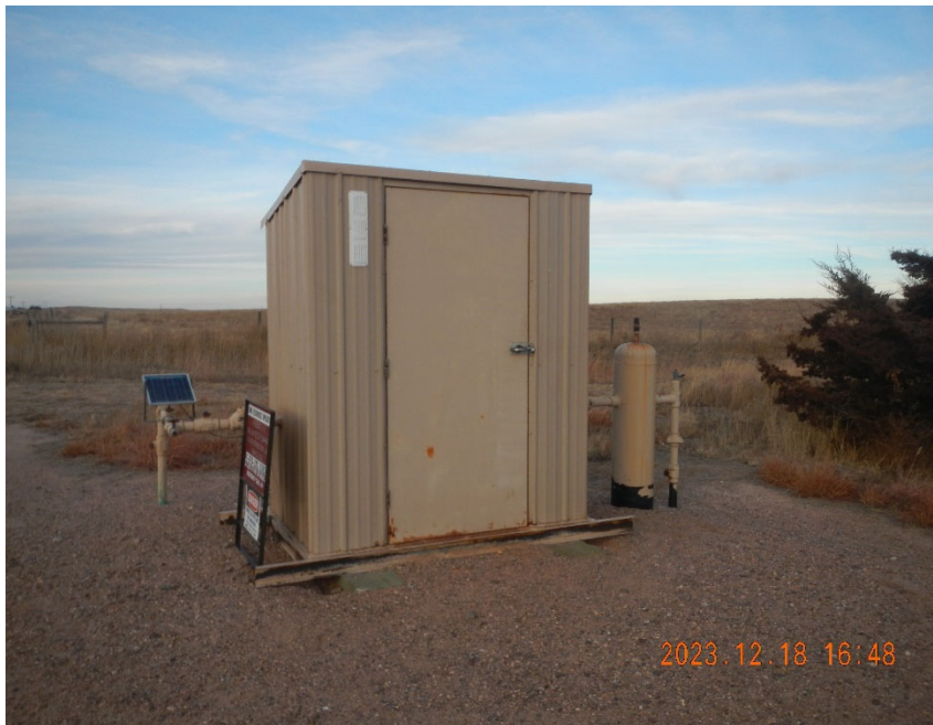
5. Meter shed and dehydrator.
