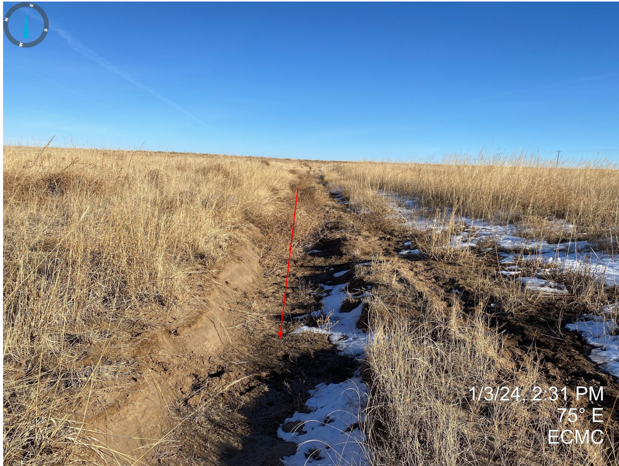
Photo 4. Erosion degradation along the access road.
