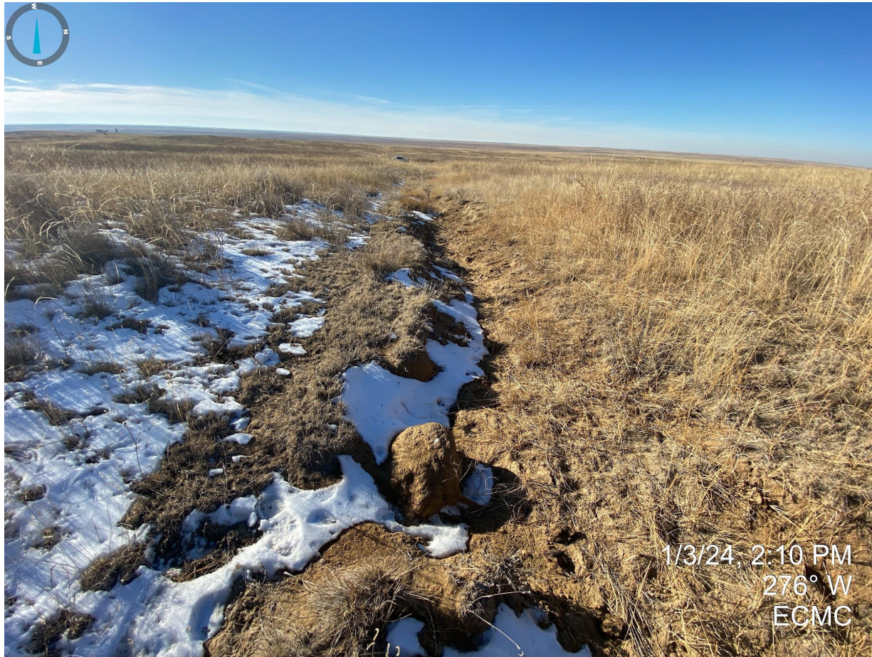
Photo 1. Stormwater erosion degradation (e.g. gully) occurring on the access road, which has not been contoured or regraded to reflect pre-disturbance levels.
