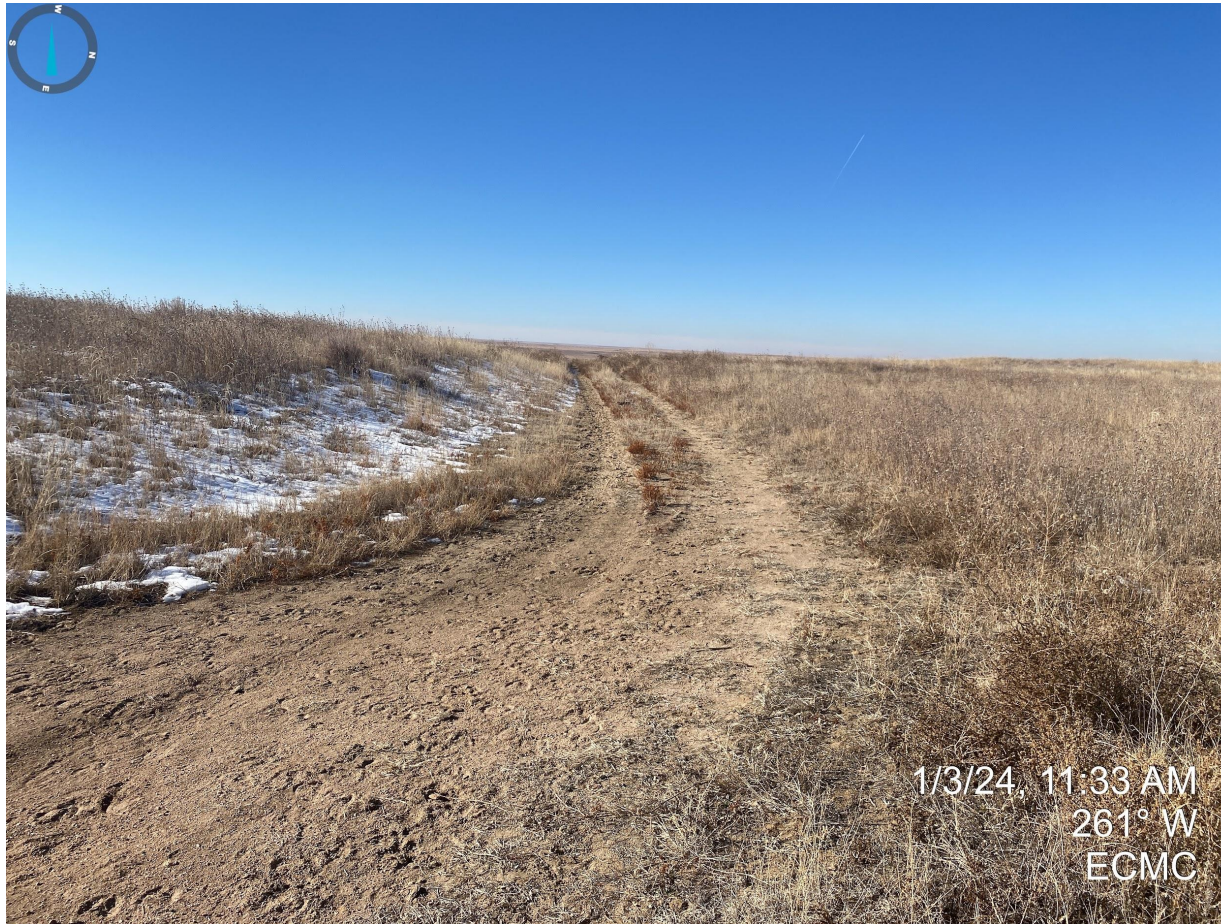
Photo 1. Facing west along the eastern part of the access road. The access road has not been reclaimed per Rule 1004; additional reclamation activities are required.
