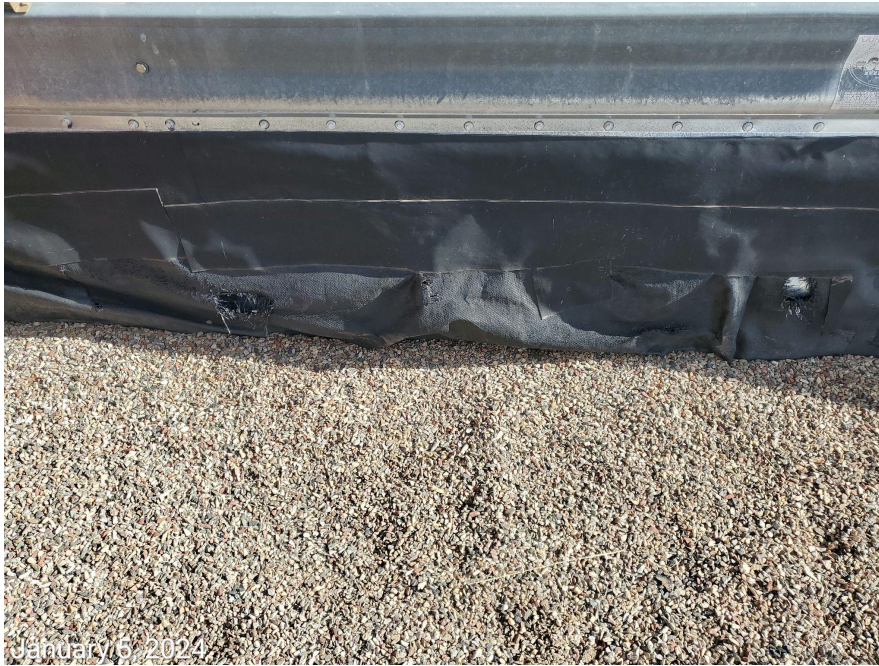
Photo 2: Photos examples showing holes/tears within secondary containment liner.
