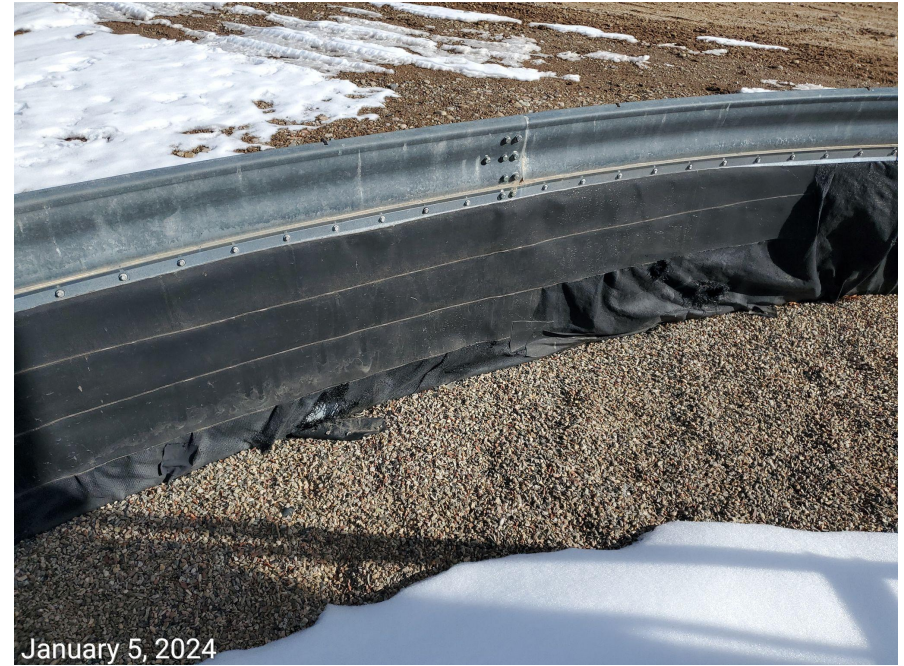
Photo 2: Photos examples showing holes/tears within secondary containment liner.
