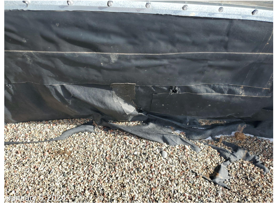
Photo 3: Photos examples showing holes/tears within secondary containment liner.
