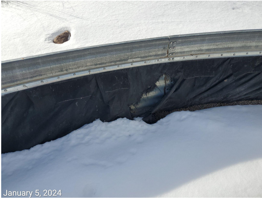
Photo 3: Photos examples showing holes/tears within secondary containment liner.
