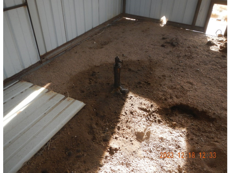
6. Riser with stained soil around it.
