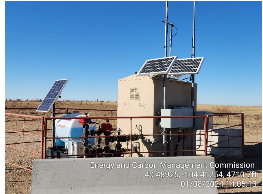
Photo 4 – Gas Lift Injection Meter House
