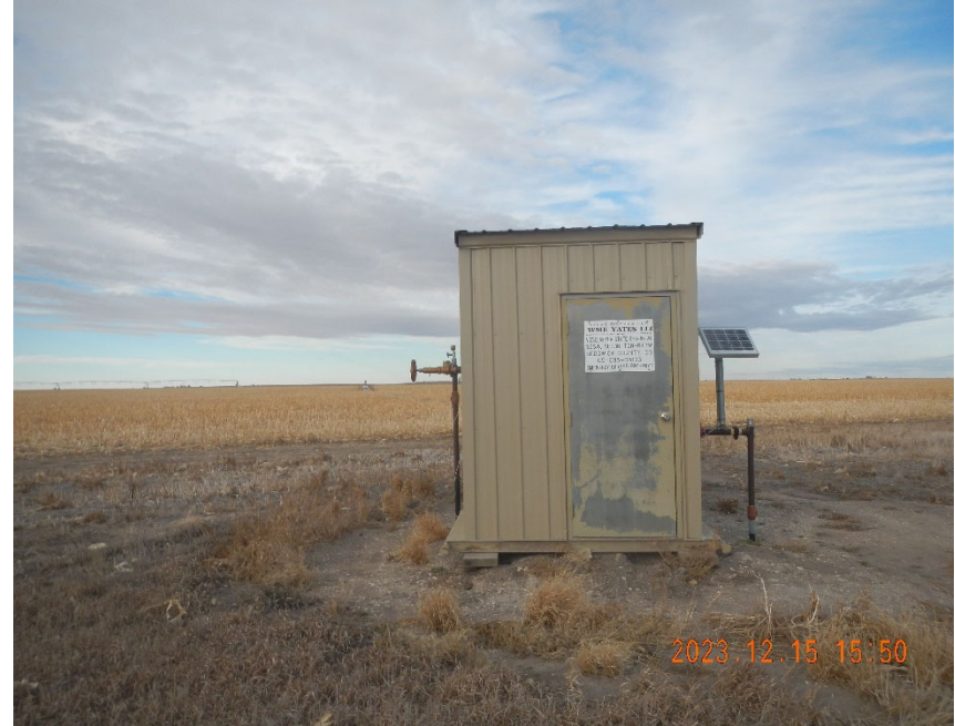
8. Meter site overview.
