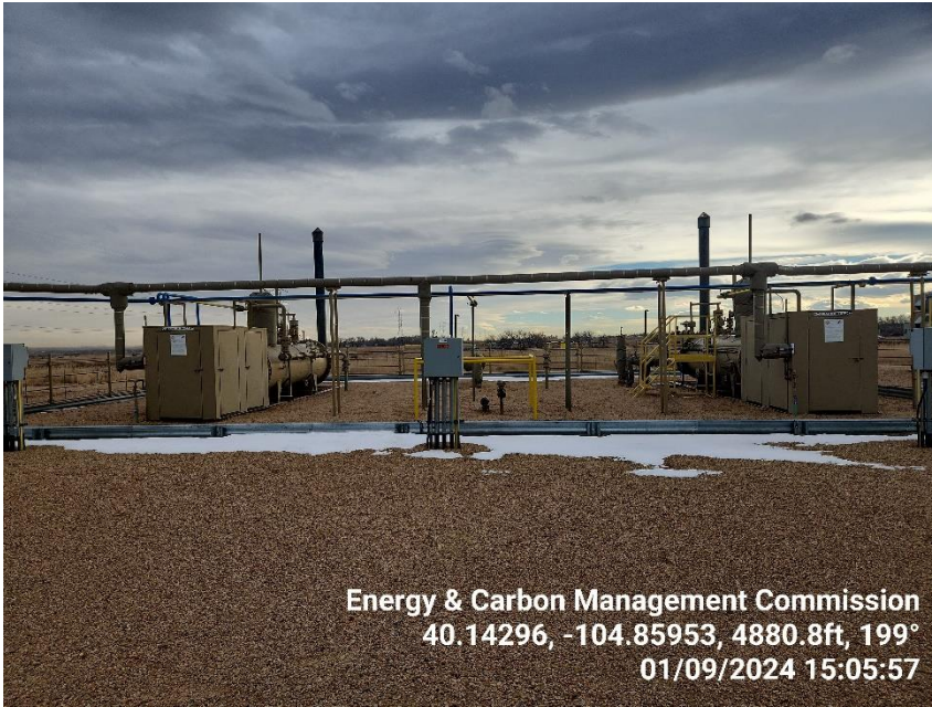
Photo 15 Horizontal Separators.
