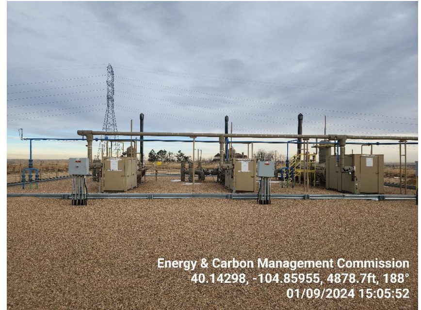
Photo 14 Horizontal Separators.
