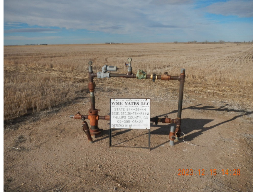
2. View of wellhead. Note capped riser.
