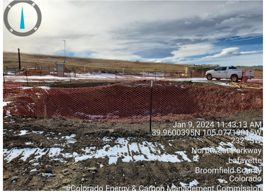
Photo 4 Open excavation around P&A well head
