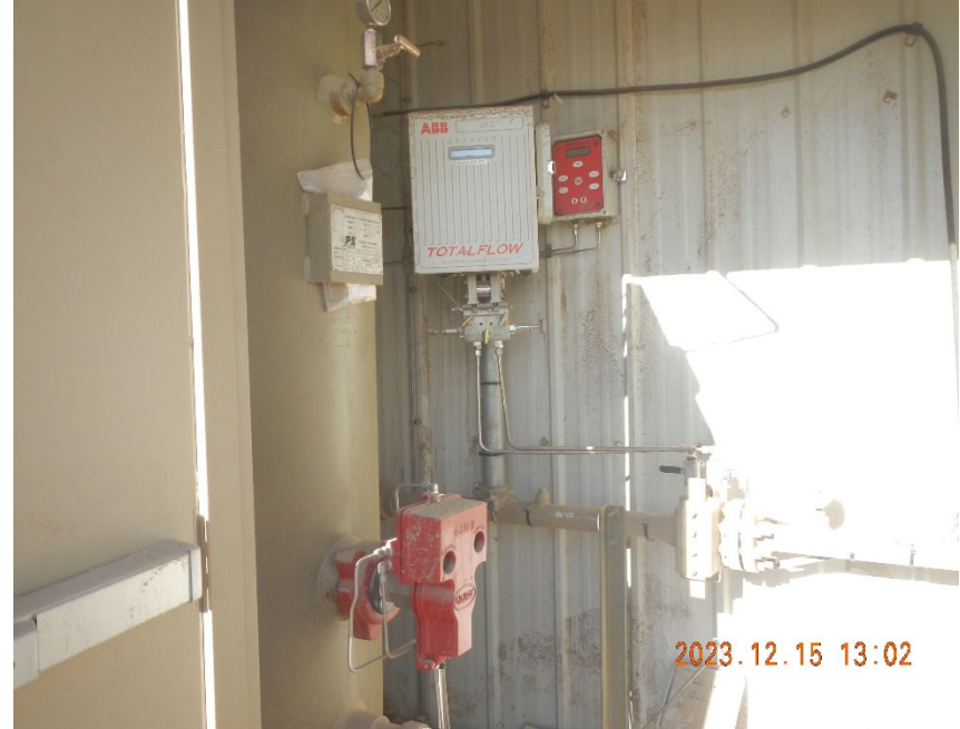
6. Vertical separator and digital gas meter inside meter shed.
