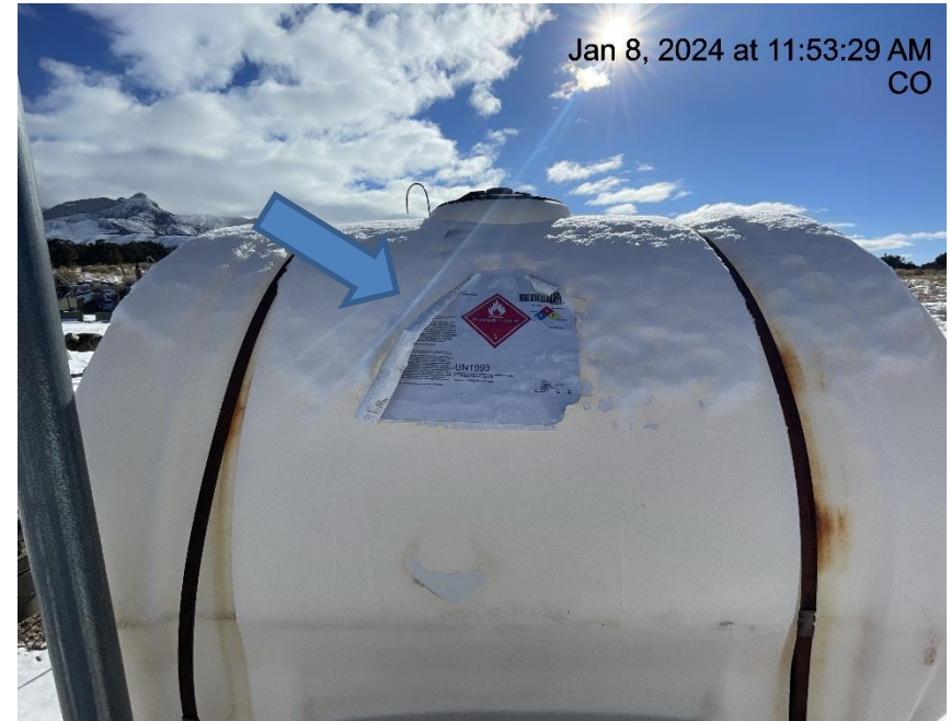
Photo # 1989 Chemical tank label peeling & illegible
