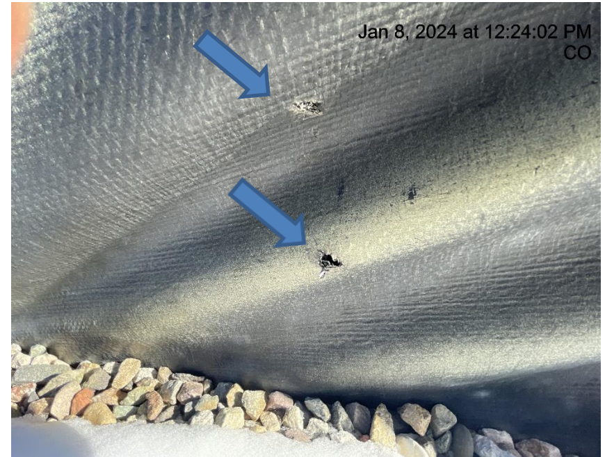
Photo # 1993 Holes in liner/liner needs maintenance
