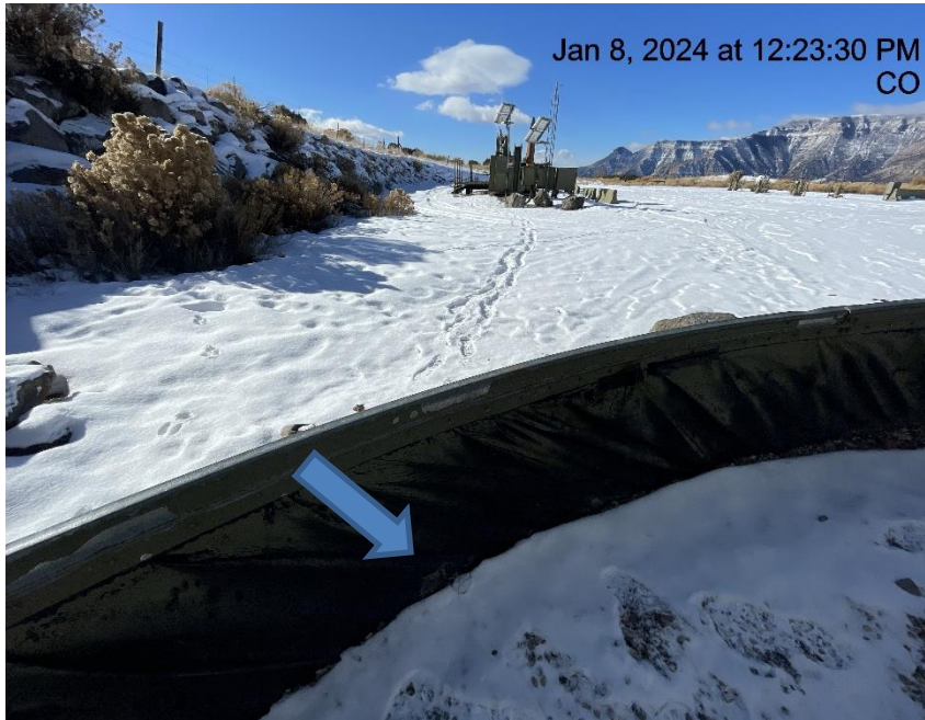
Photo # 1990 Hole in liner/liner needs maintenance
