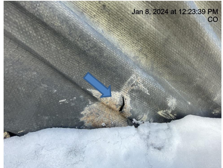
Photo # 1991 Hole in liner/liner needs maintenance
