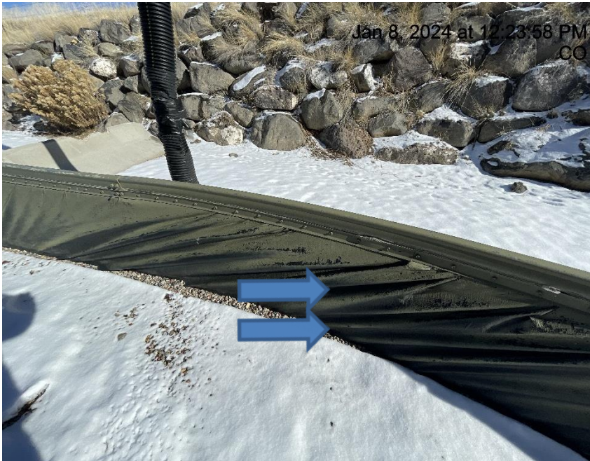
Photo # 1992 Holes in liner/liner needs maintenance
