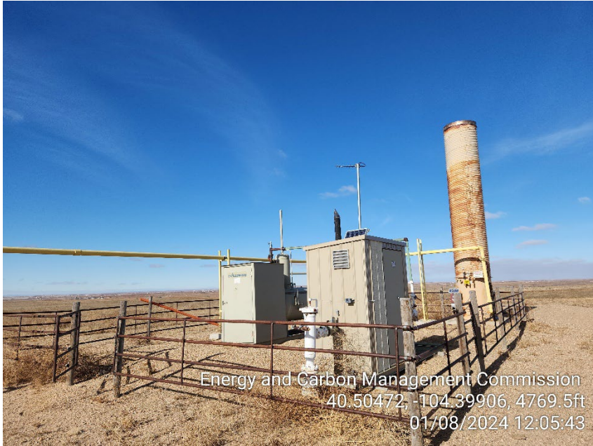
Photo 3 – Gas Meter, ECD and Separator
