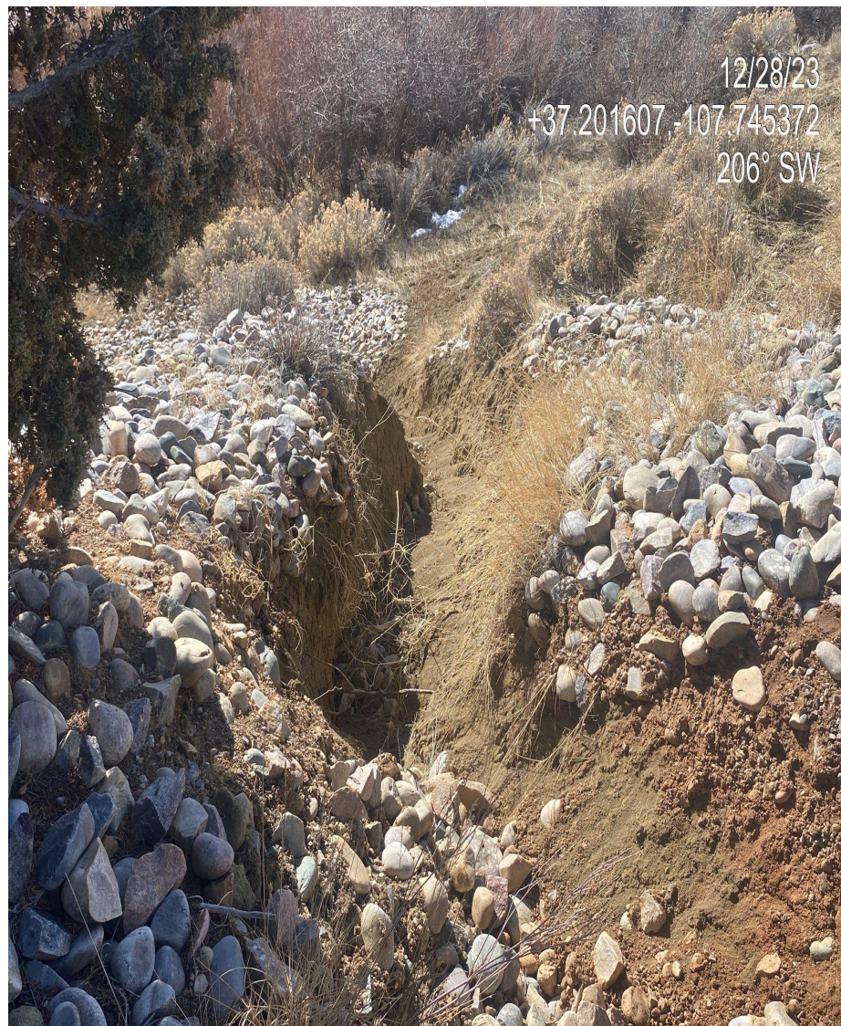
Photo 5. Severe gully erosion forming in the southern interim reclamation area.
