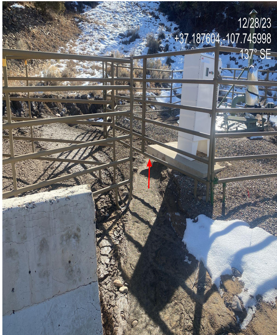
Photo 4. View of erosion on the eastern edge of the disturbance. Erosion is undercutting equipment on location and transporting sediment across the disturbance.
