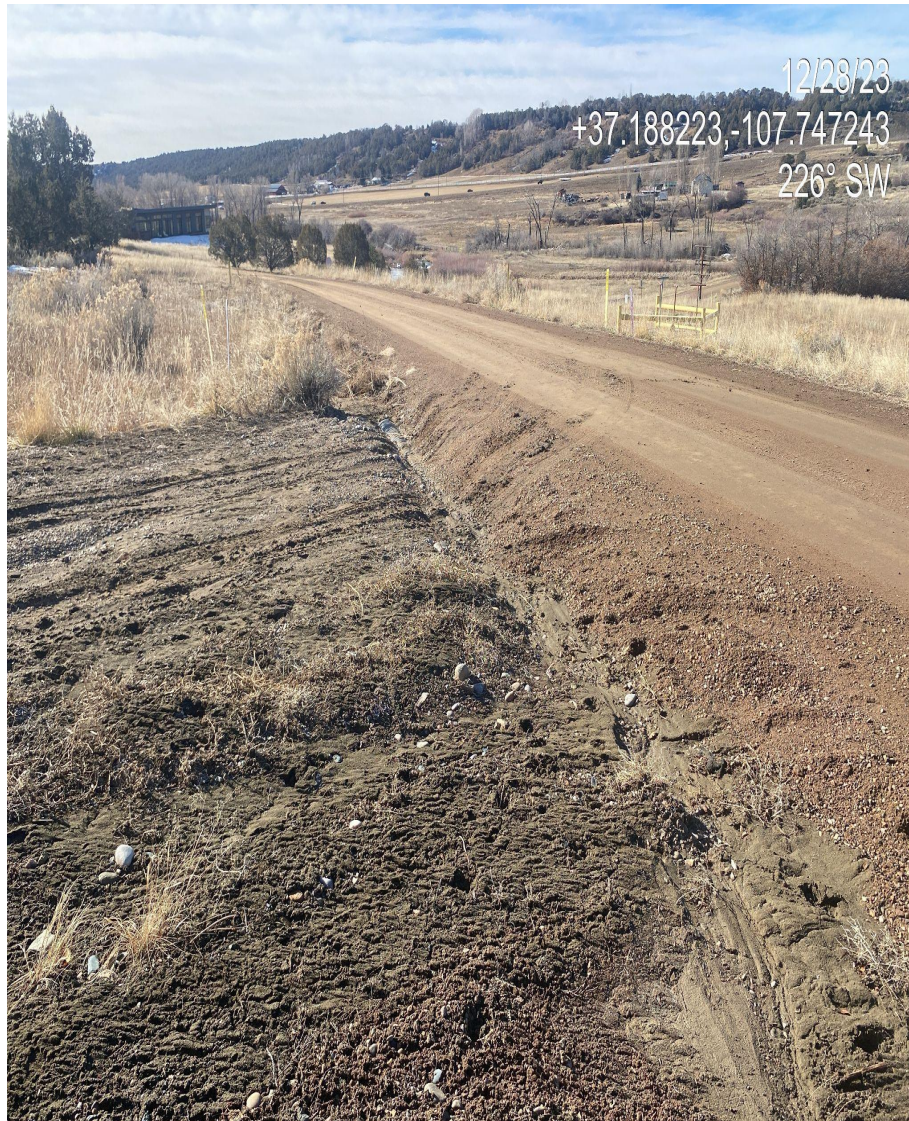
Photo 7. View of culvert at access point that is no longer functioning. Culvert is completely covered and filled with sediment, stormwater is now running over the culvert.
