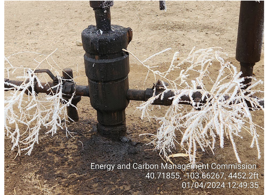
Photo 4 – Wellhead – Stained Soil
