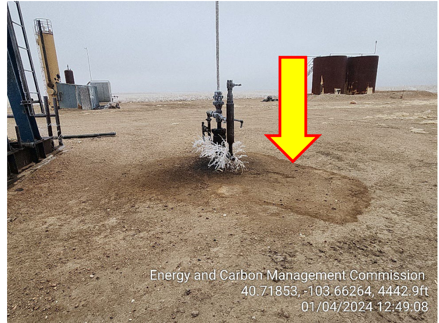
Photo 2 – Wellhead – Stained Soil
