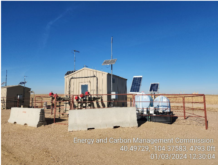
Photo 1 – Gas Lift Injection Meter House
