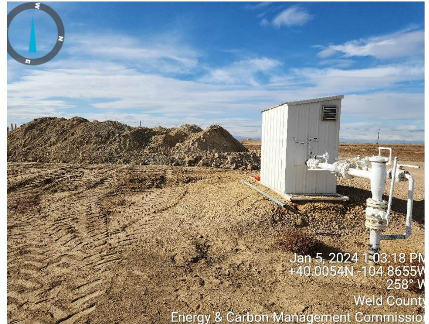
Photo 8 meter run and launcher
