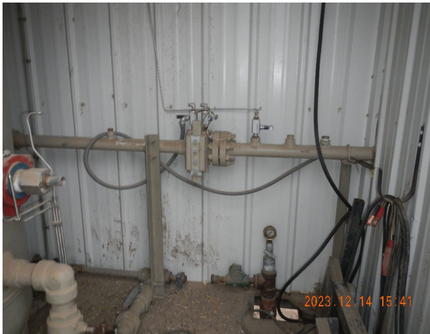
5. Vertical separator and flowline with gas meter removed.
