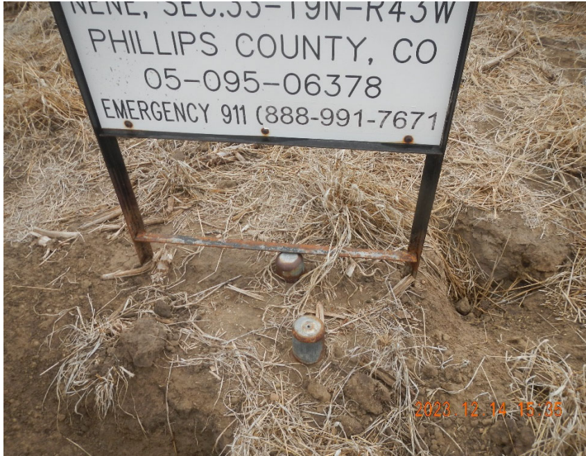
3. Capped flowlines at wellhead.
