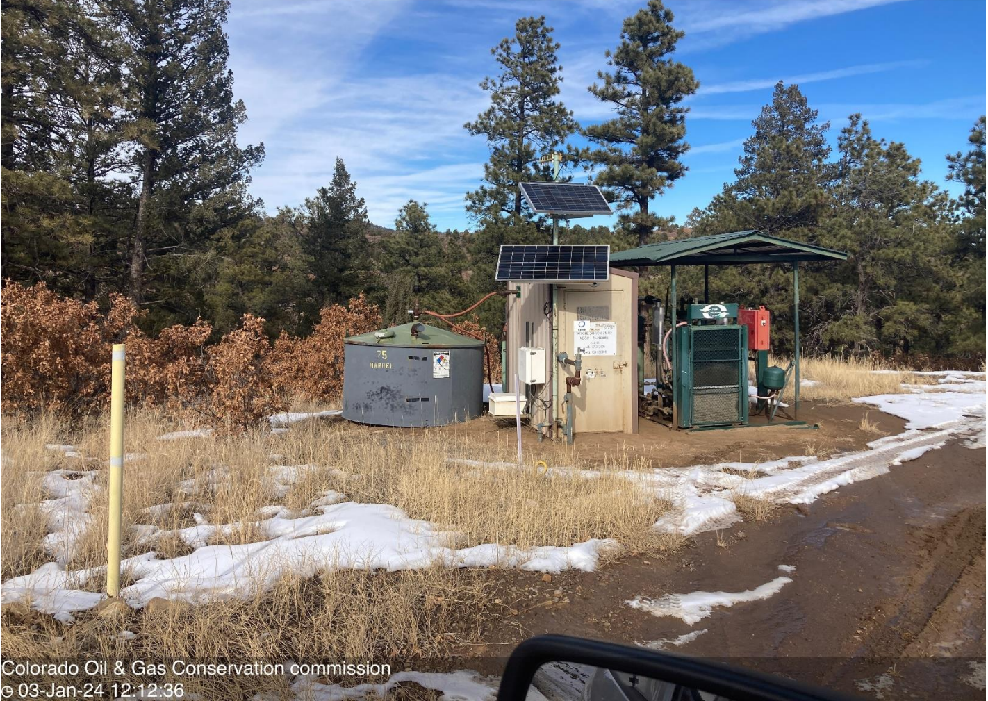
PHOTO 4: TANK BATTERY, METER HOUSE AND COMPRESSOR.
