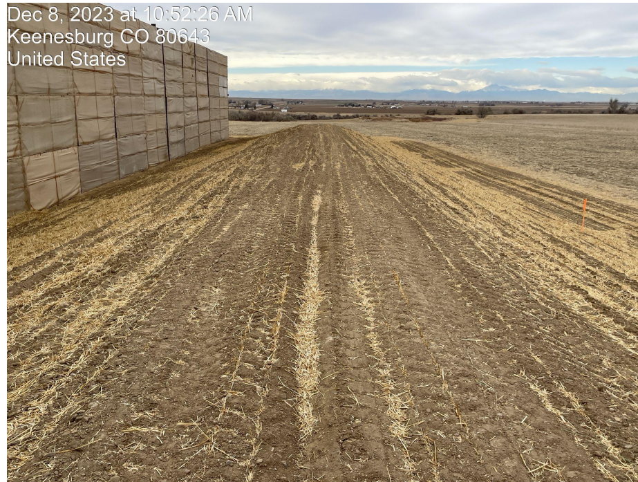
Photo 5. Photo taken on top of topsoil stockpile, lacking proper soil protection. Photo taken facing north
