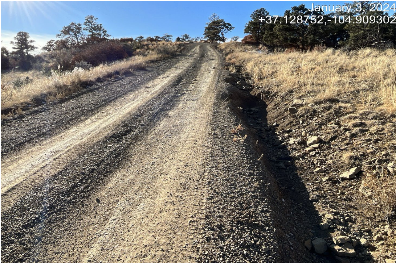
Photo 1. This area of the road side near the wellsite has eroded and needs to be repaired. .
