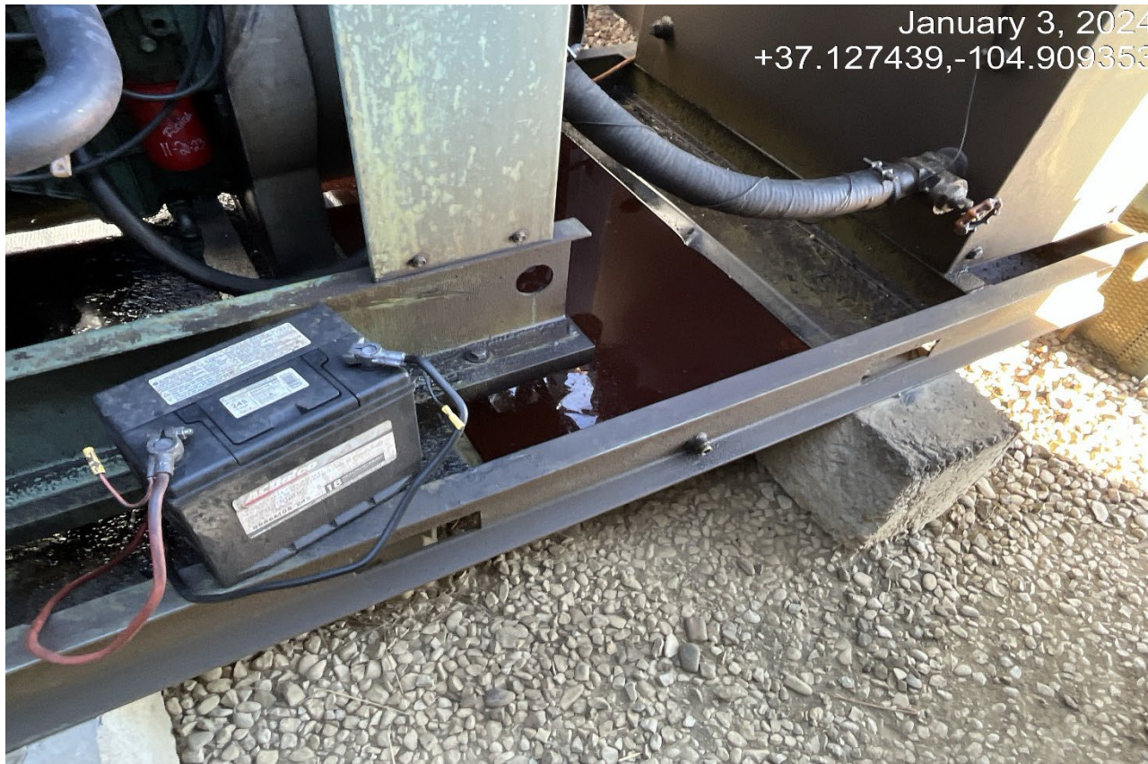
Photo 4. There is oil in the engine skid that needs to be cleaned up.
