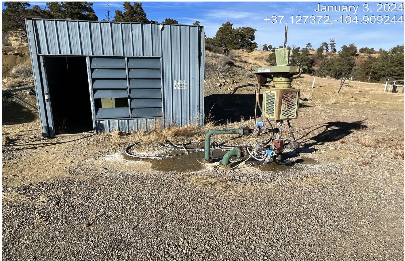
Photo 3. There is a dripping leak at the wellhead.
