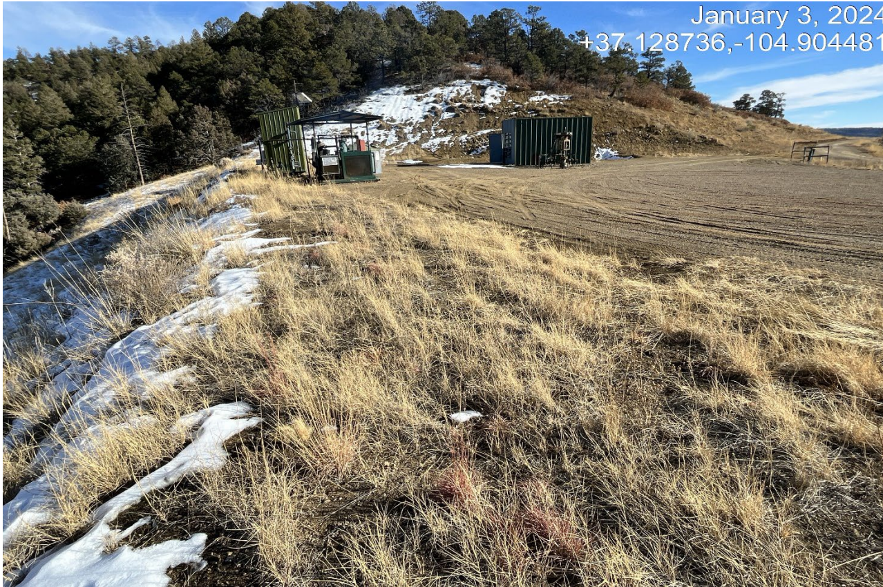
Photo 3. Facing east at the location and fill slope.
