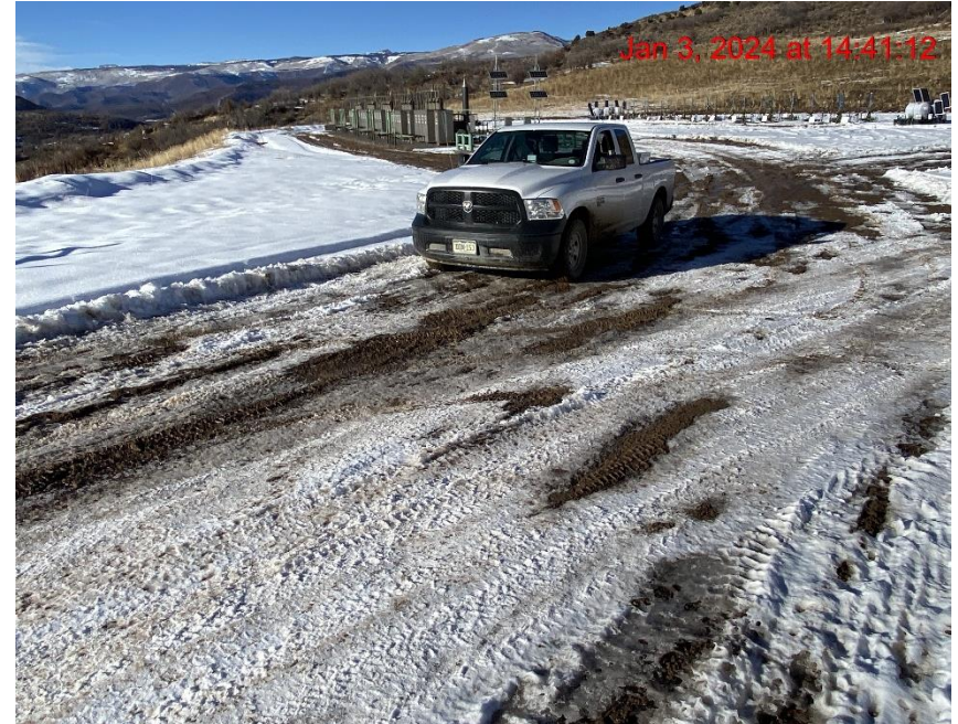
Insufficient Vehicle Tracking BMPs at Location Entrance/Exit – Photo #08492
