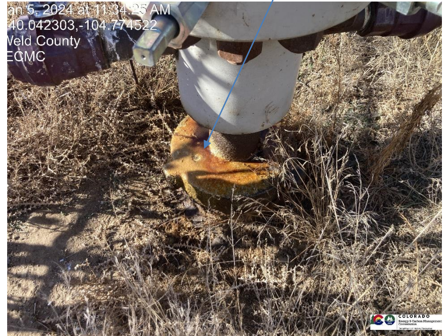
Pic 4 Leak on wellhead
