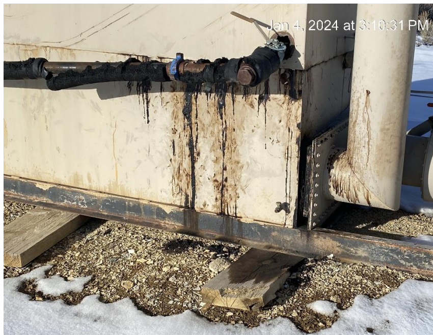
Separator leaking outside and on the ground
