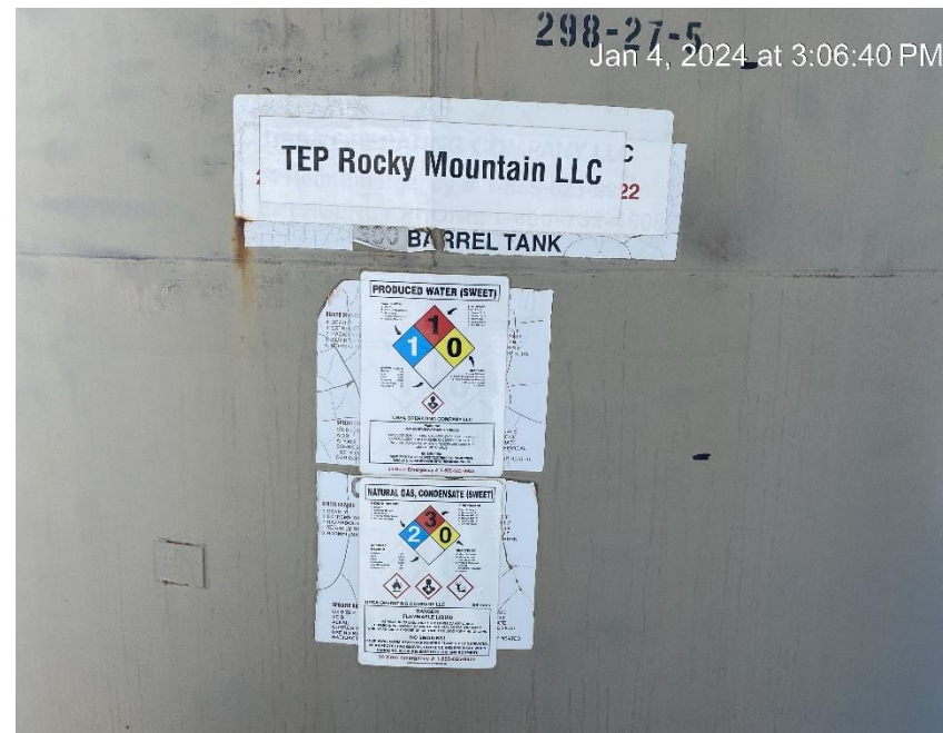
Tank labeling missing required information
