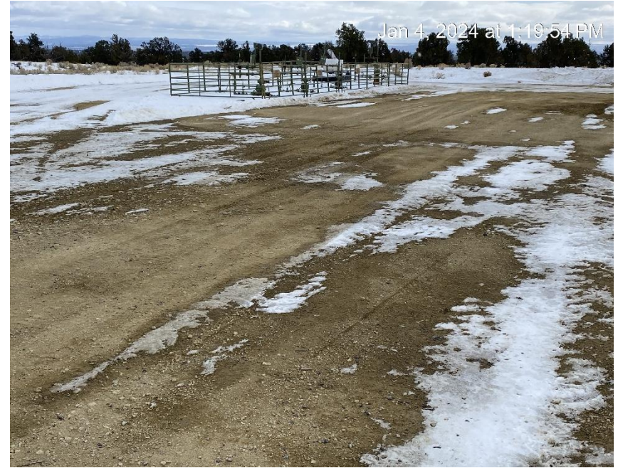
Location from Northwest corner
