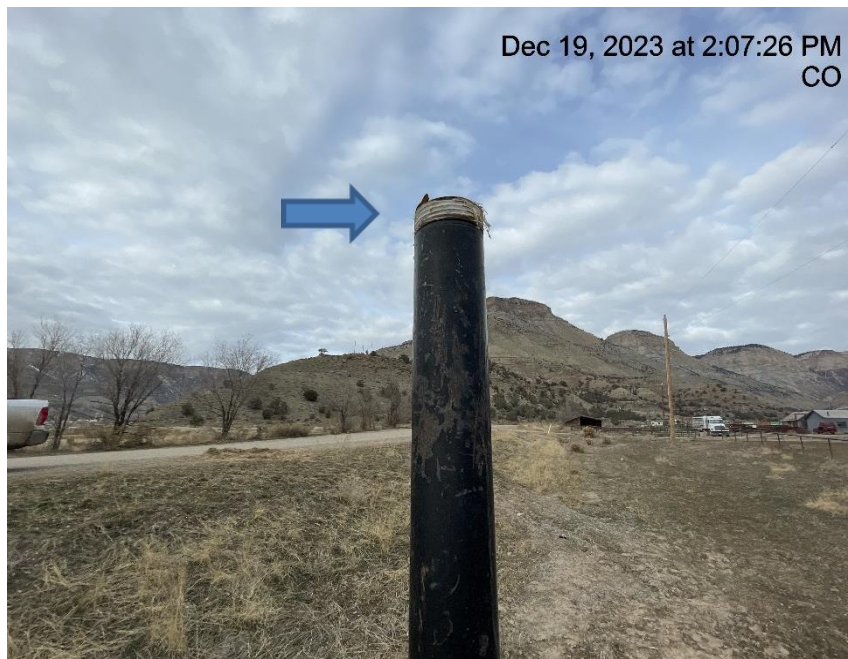
Photo # 385 From inspection 708902565 conducted on 12/19/2023 PRV vent line lacks cap
