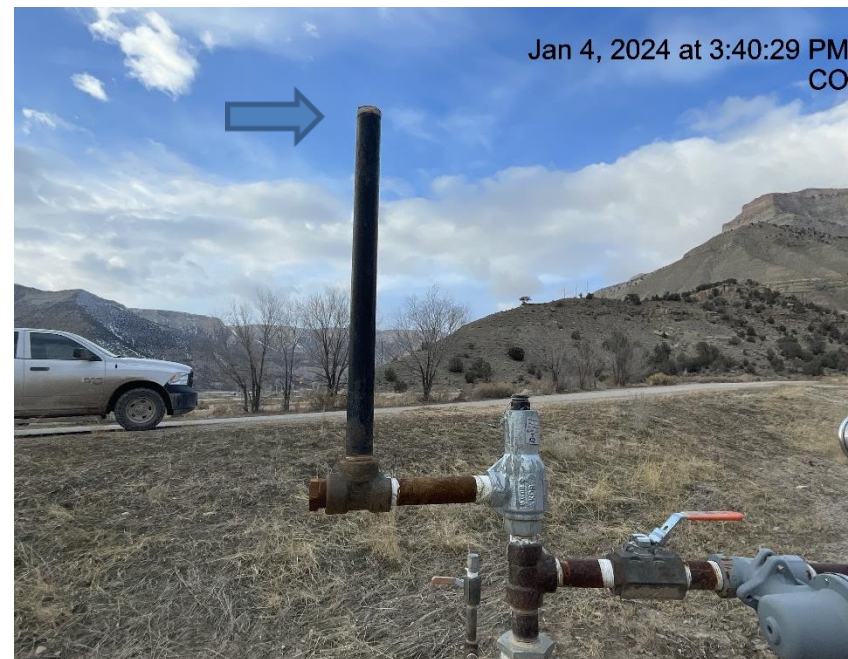
Photo # 1909 PRV vent line lacks cap
