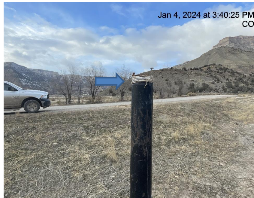
Photo # 1910 PRV vent line lacks cap
