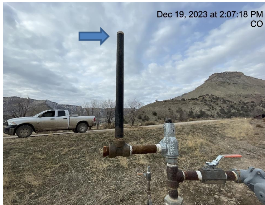
Photo # 384 From inspection 708902565 conducted on 12/19/2023 PRV vent line lacks cap
