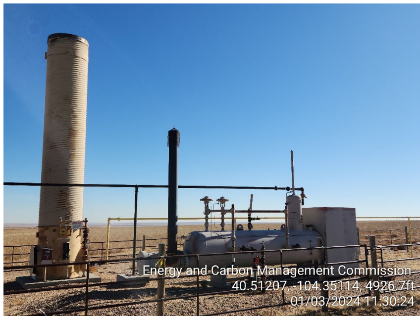
Photo 1 – ECD and Separator
