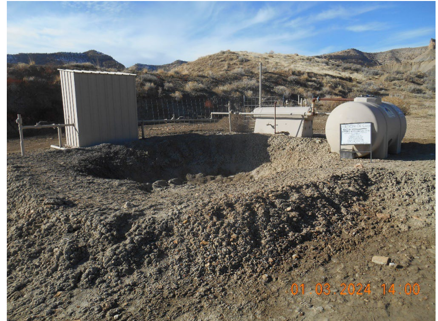
Tank Battery and Separator, Meter Housing and blowdown pit
