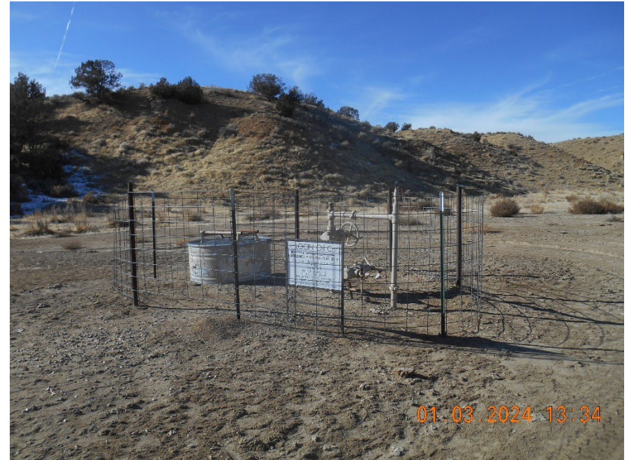
Wellhead with fencing
