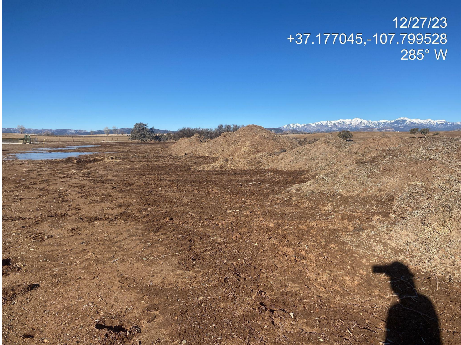
Photo 3. Large piles of unstabilized soil observed on the northern edge of the disturbance.
