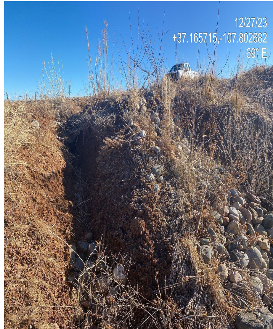
Photo 2. View of gully erosion forming in the western interim reclamation area.
