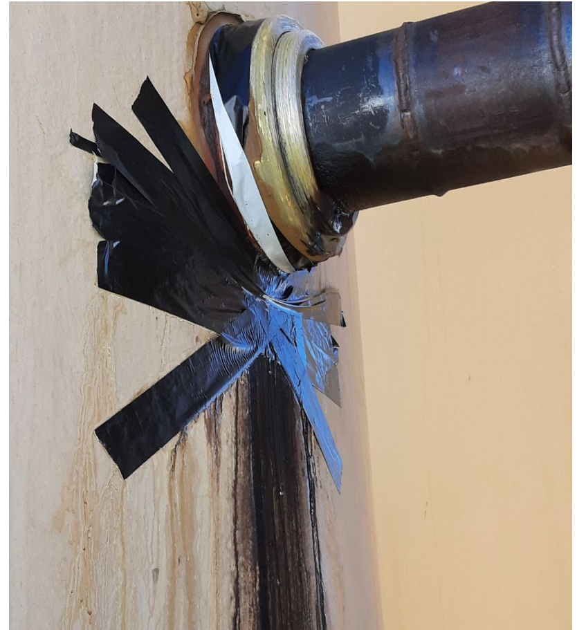
Photo 4 – Spill location and repair attempt.
