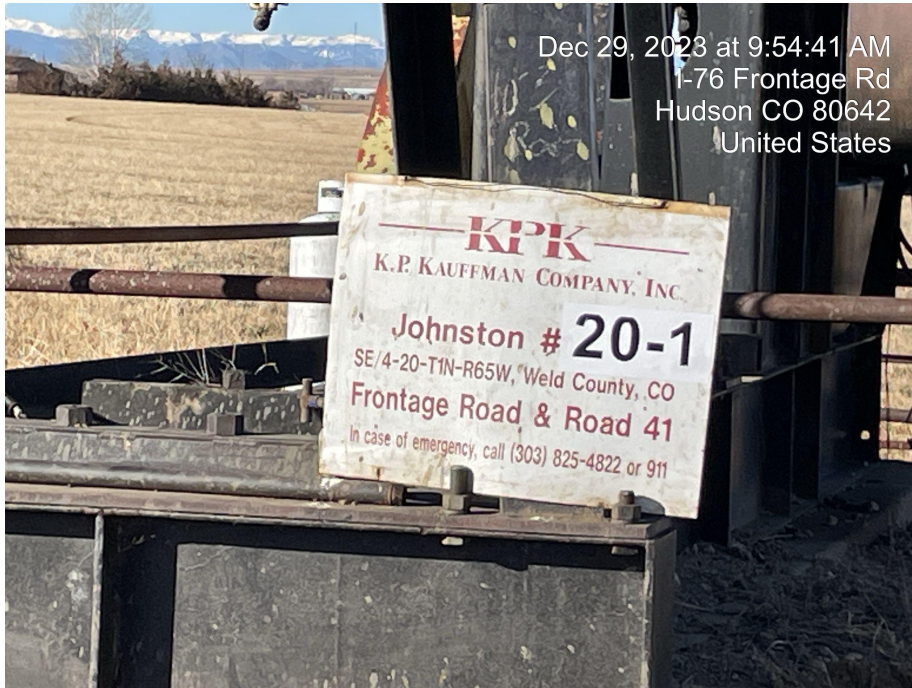
Photo 1. Photo taken of location sign at tank battery, facing northwest.
